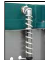
Heated option, feed pipe with frost protection heating cable wrapped around the valve
